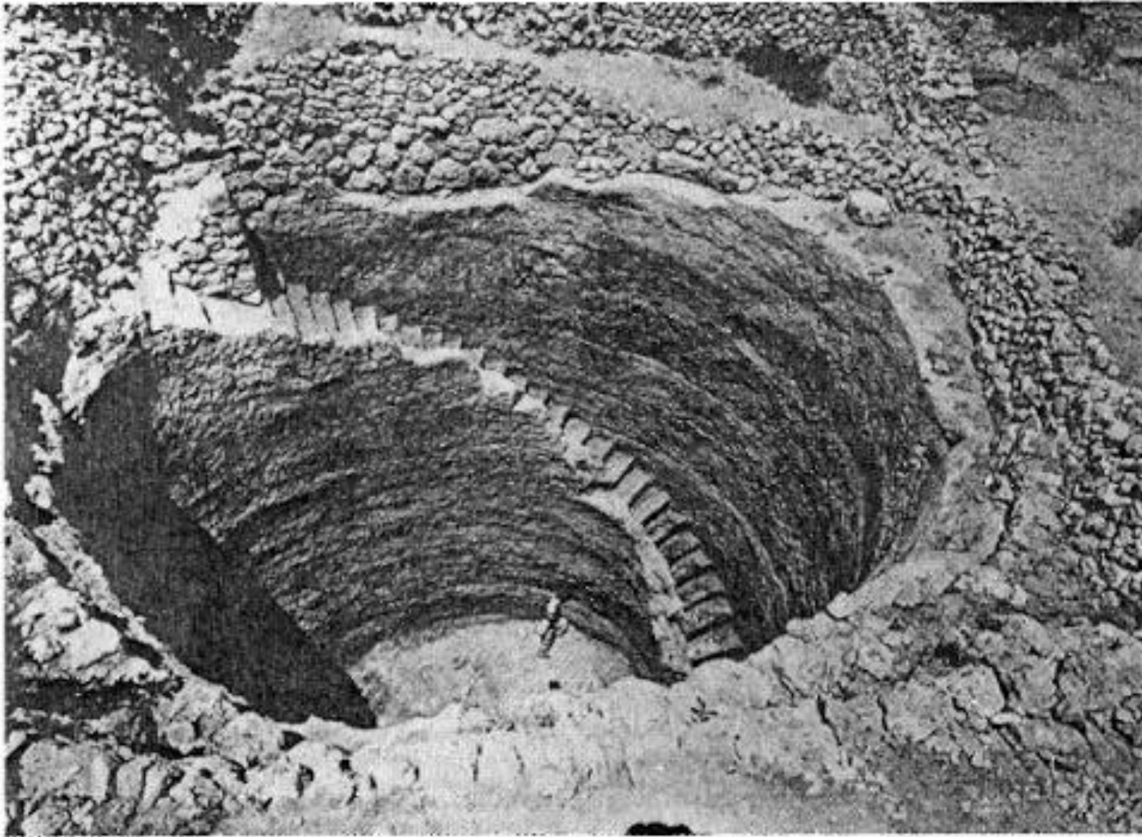
Diagram 6. Pool of Gibeon —a great water-shaft sunk into the bedrock to reach the water table.
